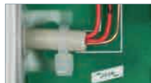
Conductor fixing by means of cable ties (DBX TC 180).
