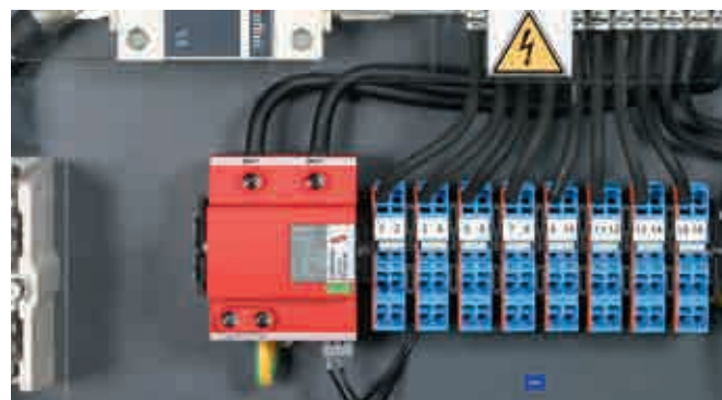
For protecting photovoltaic inverters against surges and even direct lightning strikes. For use in accordance with IEC 60364-7-712 (Installation of photovoltaic power supply systems).
