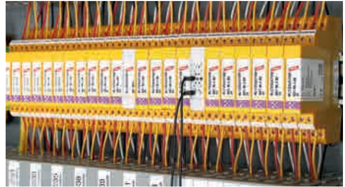
BLITZDUCTOR XT with an earthing module (grey). The lines can be tested by means of the measuring module (grey with lines) without disconnecting the terminals.
