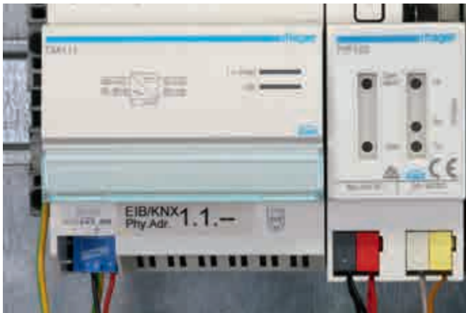
Protection of a KNX power supply unit by means of a BUSstector surge arrester mounted in the bus terminal slot.
