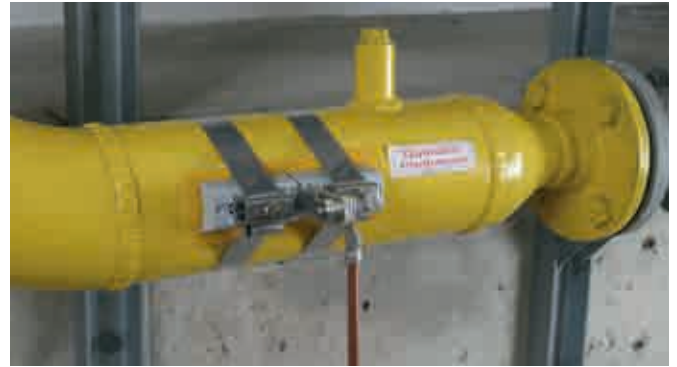
Pipe clamp for electrical contacting of pipes in explosion-hazardous areas for implementing of lightning equipotential bonding according to IEC/EN 62305-3
