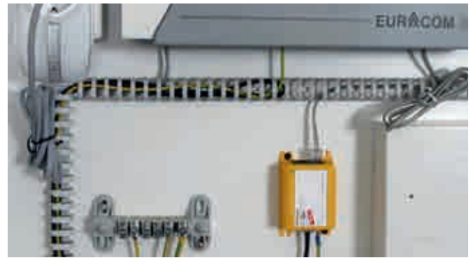
Surface-mounted surge arrester for telecommunications terminal equipment as well as telephone systems with RJ plug.
