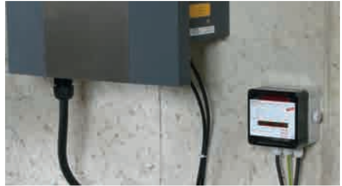
For protecting low-voltage consumer's installations against surges. For use in accordance with IEC 60364-7-712 (installation of photovoltaic power supply systems).
