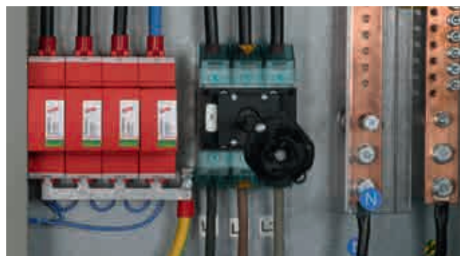
Single-pole surge arrester with integrated “Lifetime Indication” early warning system. For protecting low-voltage consumer’s installations from surges. For installation in conformity with the lightning protection zone concept at the boundaries from O_B - 1 and higher.
