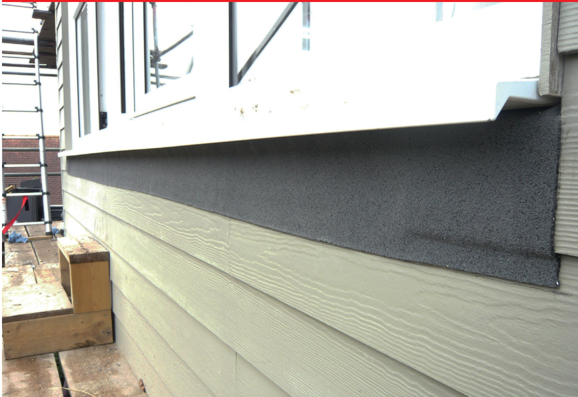
Left image Detail of Ubiflex window flashing
