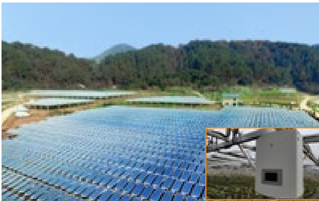
Zhejiang Dajie Agricultural-photovoltaic hybrid PV plant 3MW
