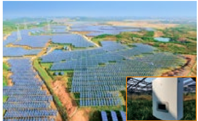
Zhejiang Hangbu Agricultural-photovoltaic hybrid PV plant 30MW
