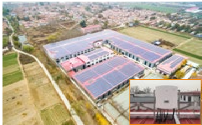
Shandong YUELONG 3.5MW
