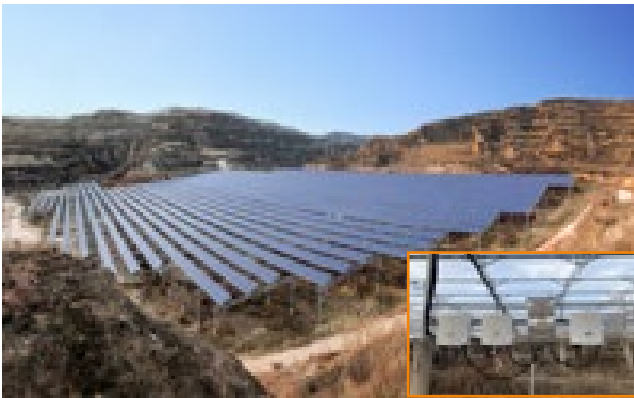
Shanxi Lvliang ZhongYang poverty alleviation PV Plant 10.3MW
