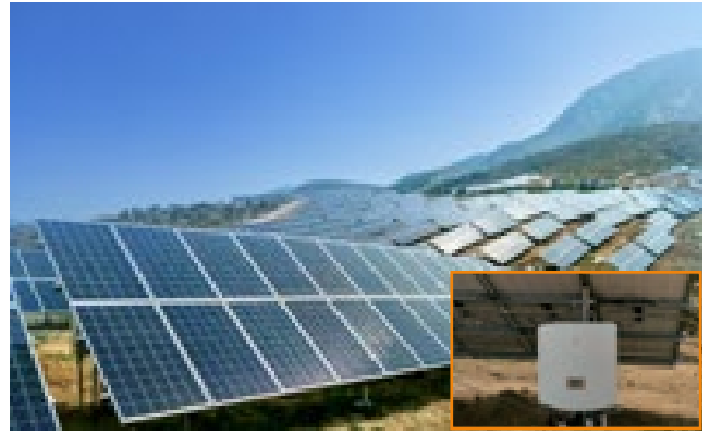
Liaoning Yingkou Jiuzhai PV plant 20MW
