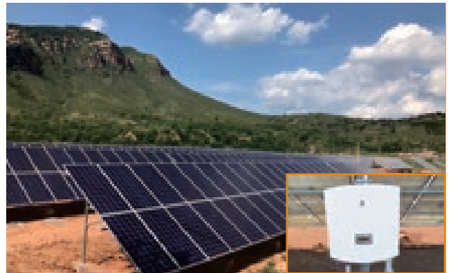
Shanxi Xiyang poverty alleviation PV Plant 7.2MW
