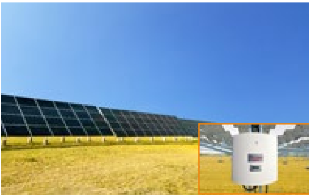
Huaneng Yimin surface mine PV plant 20MW
