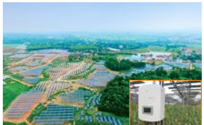
Quzhou Qinghu Agricultural-photovoltaic hybrid PV plant 20MW
