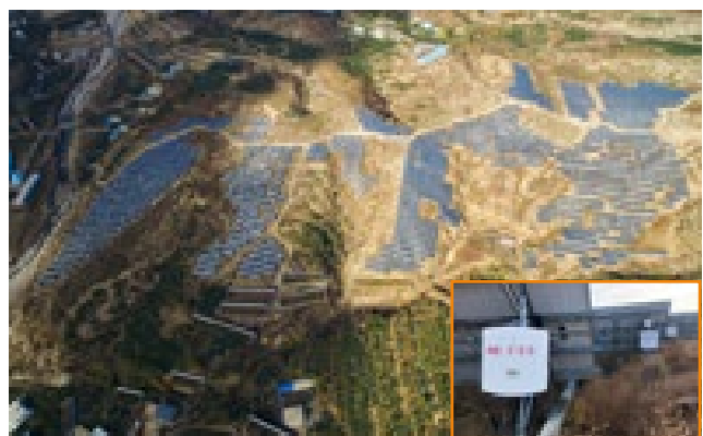
Liaoning Jiuzhai Gaizhou PV plant 20MW
