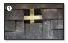
Place the bottom section of the ERIC-TILE (A) in place of the previously removed tile situated directly over the rafter. Fix with supplied clout nails x2 (D). Make sure the EPDM strip is positioned correctly. (shown on right).
