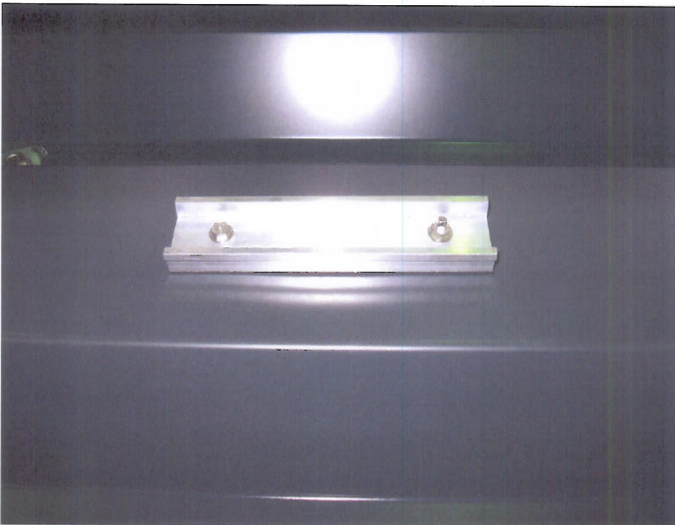
Fig. 4: clamp base fastened on the trapezoidal steel sheet with the SFS drilling screws on the left: head cap already untightened
