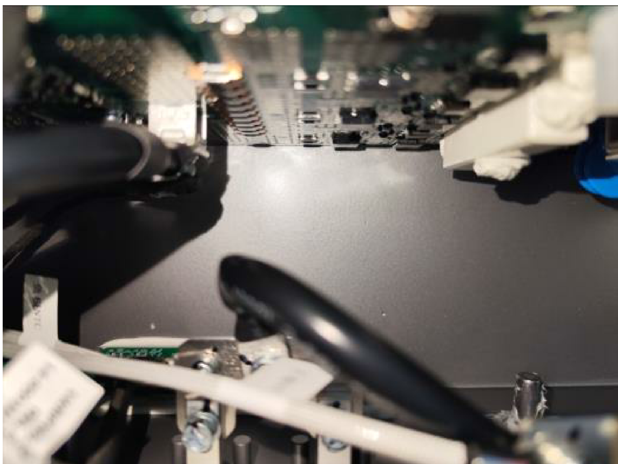
Fig.R02.6 After the test no water inside
