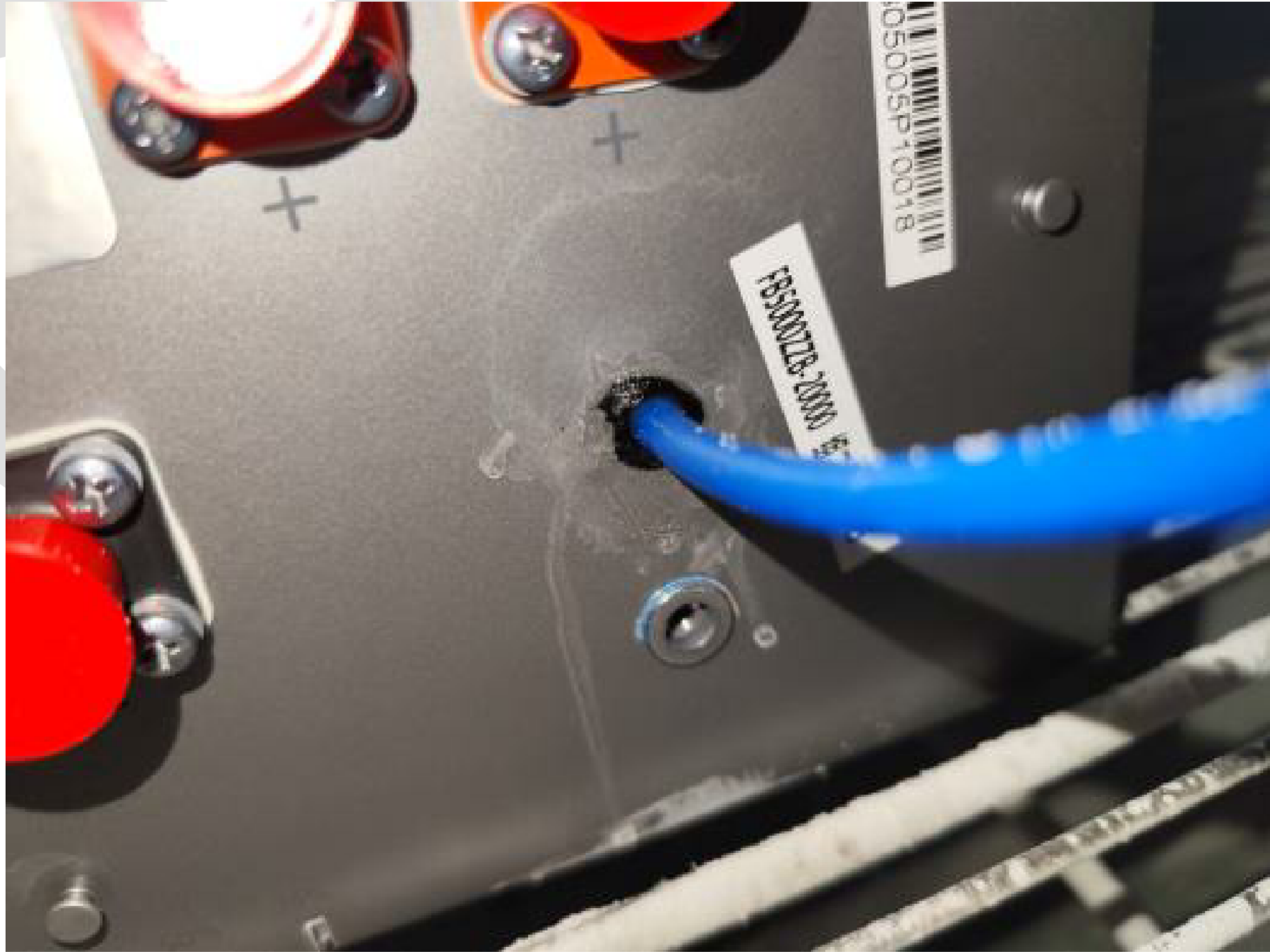
Fig.R01.2 Pumping position
