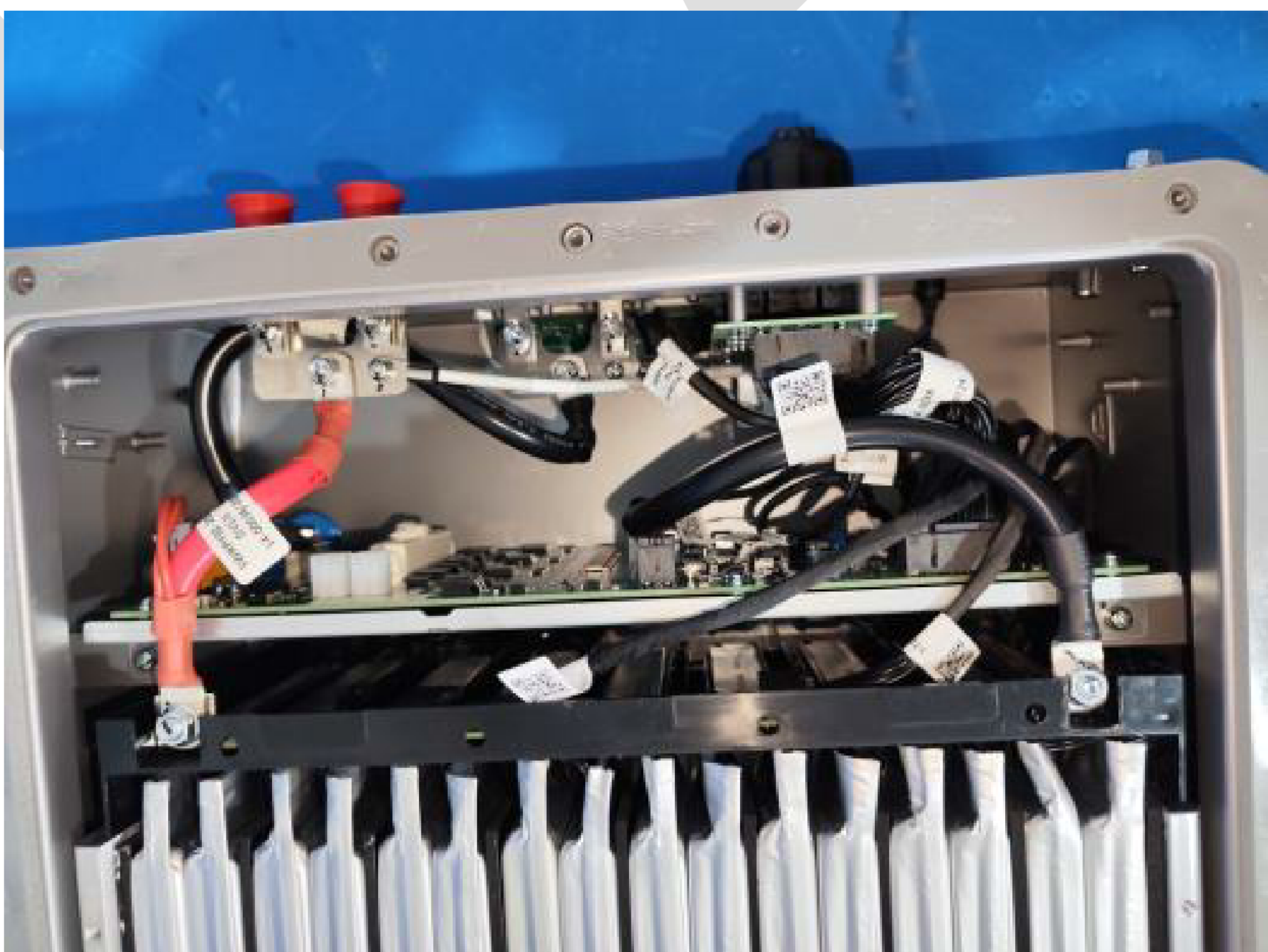
Fig.R02.5 After the test no water inside
