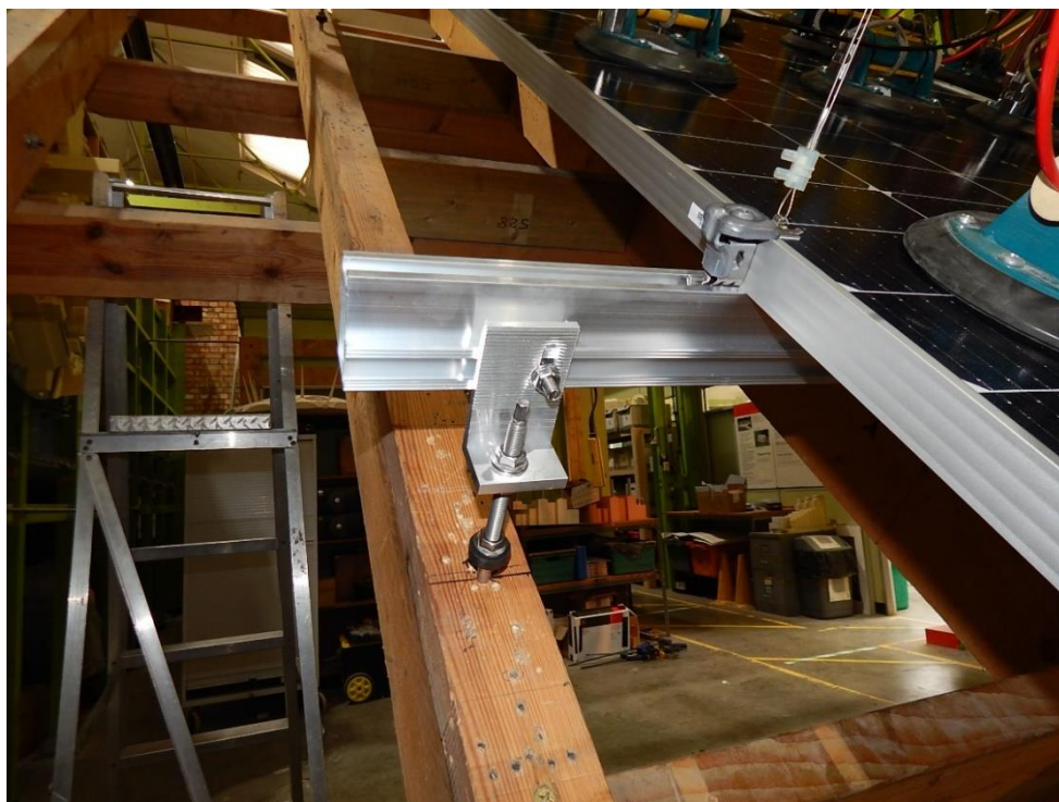
Figure 6. Installation of the offset hanger bolt to the BRE test rig.
