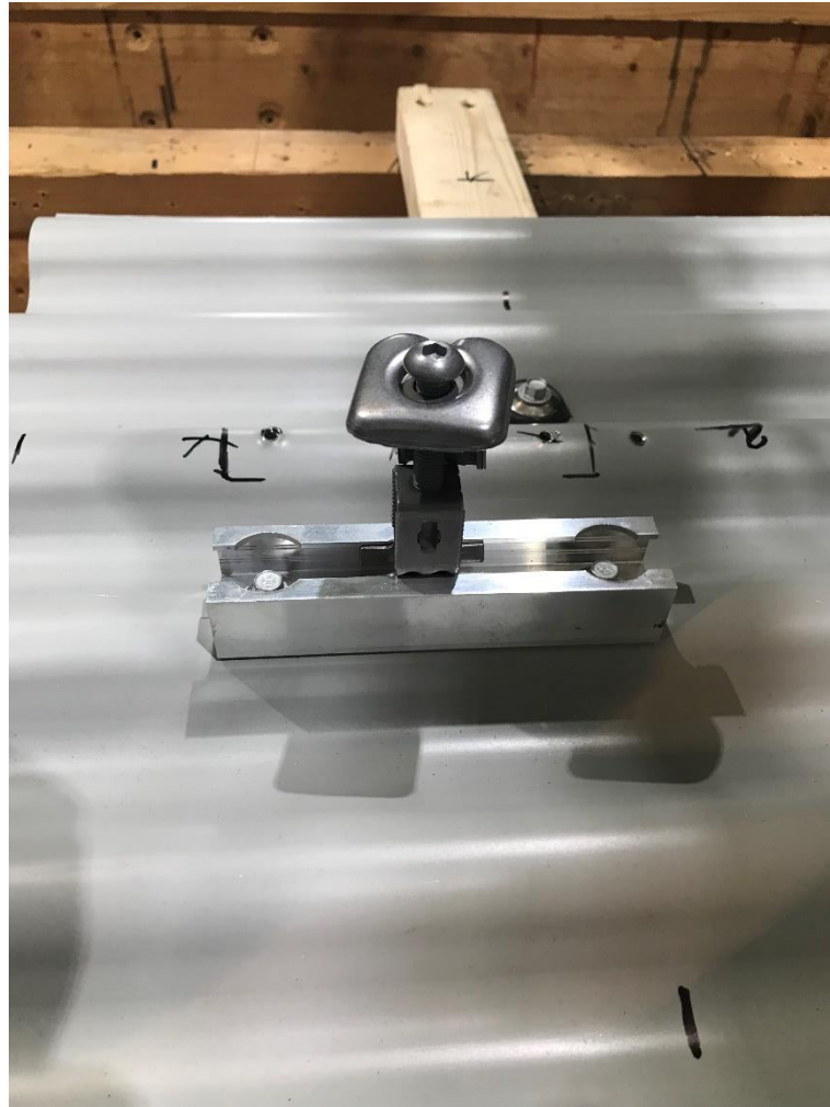
Figure 8. Installation of the Metasole bracket to the BRE test rig.
