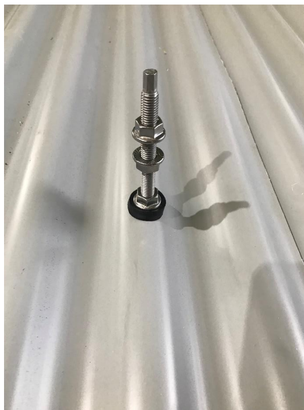
Figure 7. Hanger bolt installed prior to test.
