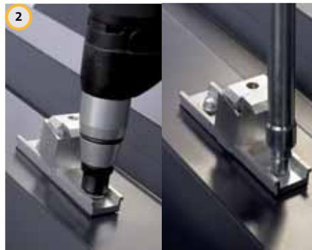
2 Installation of the lower clamp base
